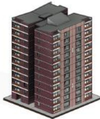
EXISTING SOUTH WEST
